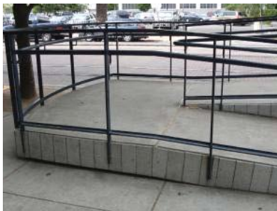
Figure 22. Ramp with continuous handrails.
