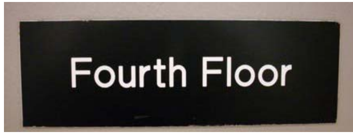
Figure 17. Accessible sign showing light characters on a dark background.
