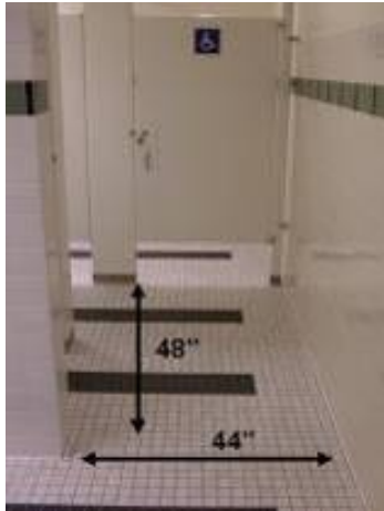
Figure 35: Restroom clear floor space on the path of travel to the toilet stall.
