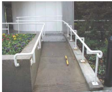
Figure 21. Accessible ramp with edge protection.
