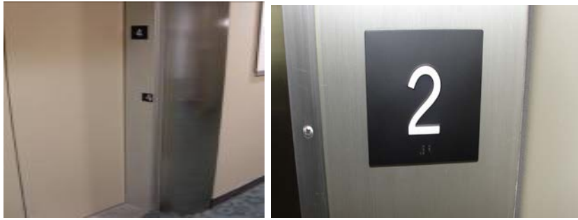
Figure 26. Signs within the door jamb or frame of the elevator landing indicating the floor designation.
