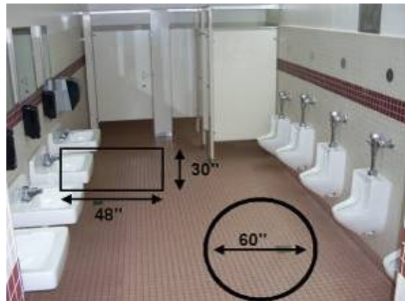
Figure 32. The inside of a restroom showing floor space measurements.
