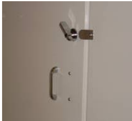
Figure 34. Restroom door with an accessible handle and flip over style hardware.
