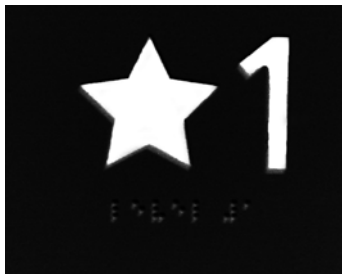
Figure 27. A raised five-point star shown on the left side of the main floor number.
